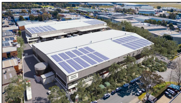
373 Horsley Road, Milperra (Under Construction)
